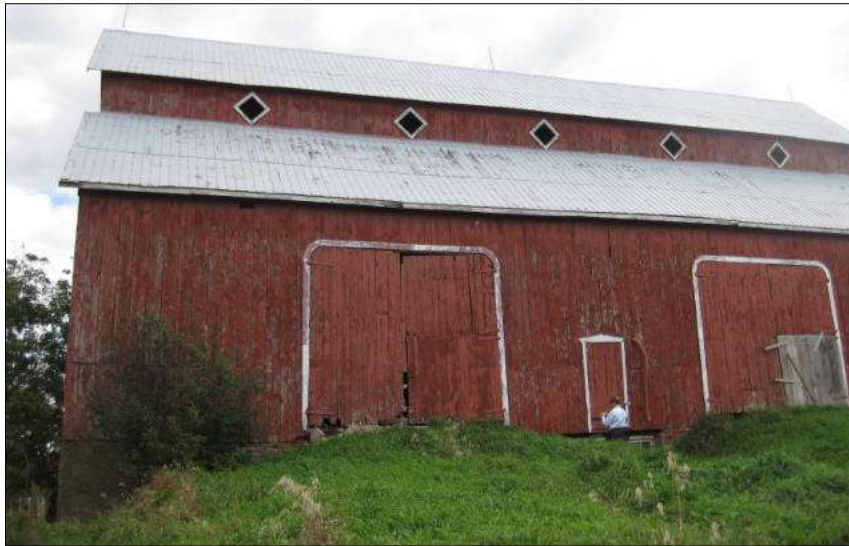
Figure 12: Bradley/Craig Barn north elevation showing earth mounds leading to double doors with a centre man door, monitor roof line, wood cladding, and diamond-shaped clerestory windows.
