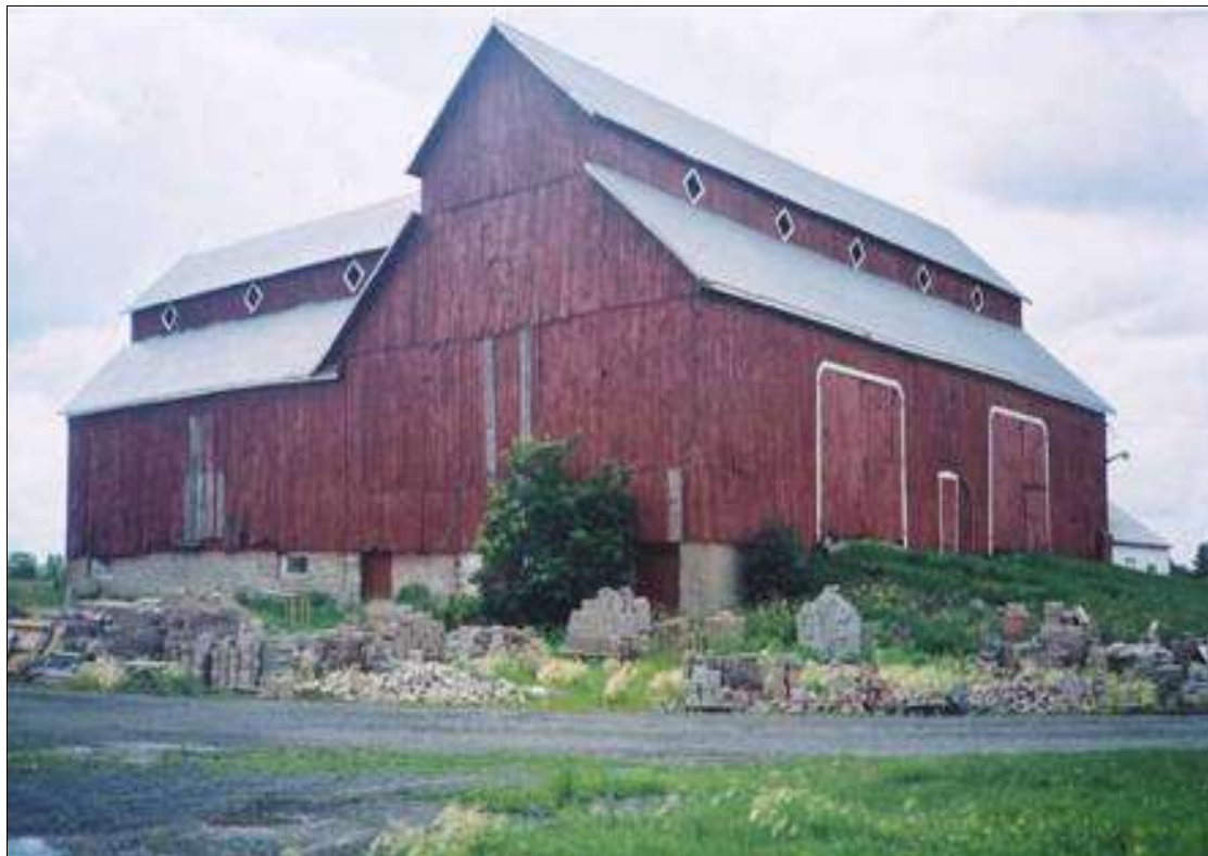
Figure 13: Northeast Elevation of the Bradley/Craig Barn in 2003. This view shows the extension, monitor roof lines, stone foundation, wood cladding, diamond-shaped clerestory windows, and raised two-bay barn plan. This is an important contextual view establishing the scale of the barn and the manner, in which it is situated. Credit: Carol Ruddy and City of Ottawa Designation Report.
