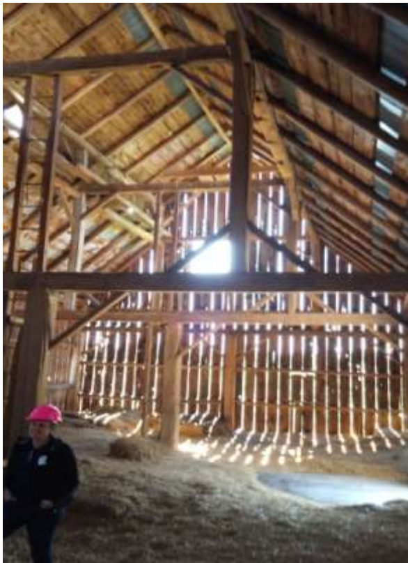
Figures 14, and 15: Interior views of the barn 2015. "Gaps between barn boards are not the result of carelessness but were deliberately included to provide for air circulation. They also admitted filter light and an empty barn in June just before the first hay is garnered, can inspire thoughts of medieval castles 2 ." Figure 16: The view of the lower level tail documents a slightly smaller footprint that served as the nursery for calves, the bull, and work horses. Credit: Commonwealth/Richcraft
