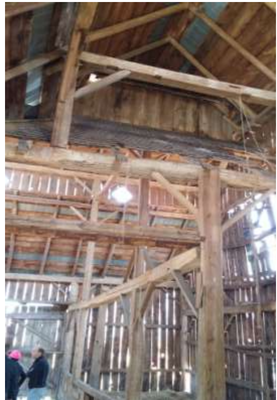
Figures 14, and 15: Interior views of the barn 2015. "Gaps between barn boards are not the result of carelessness but were deliberately included to provide for air circulation. They also admitted filter light and an empty barn in June just before the first hay is garnered, can inspire thoughts of medieval castles 2 ." Figure 16: The view of the lower level tail documents a slightly smaller footprint that served as the nursery for calves, the bull, and work horses. Credit: Commonwealth/Richcraft
