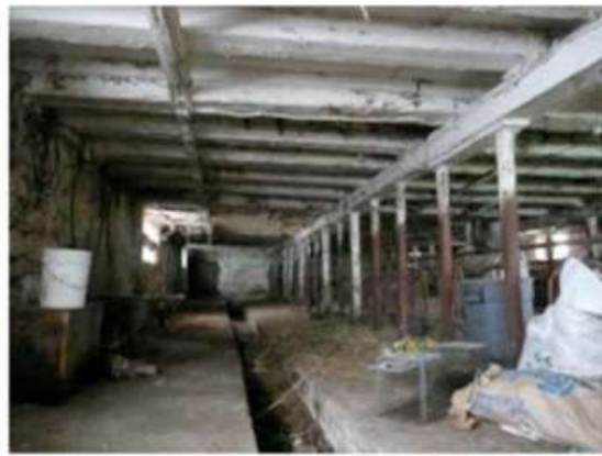
Photo 16: Barn lower stall area. Note manure removal system.
